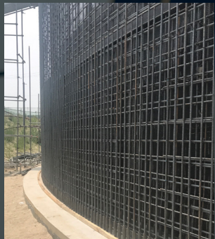
Impossible to lap splice area
